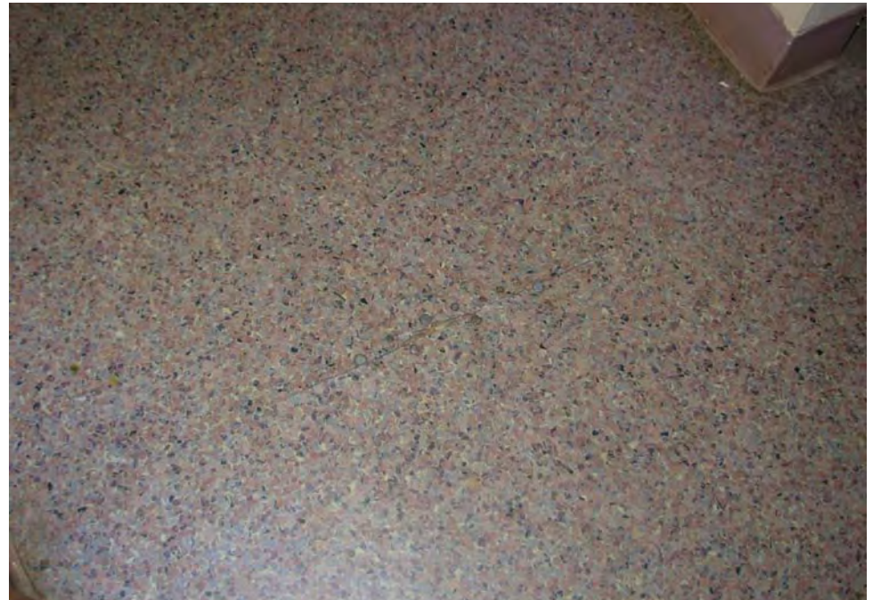
12. Unit vinyl flooring seam separation - trip hazards
