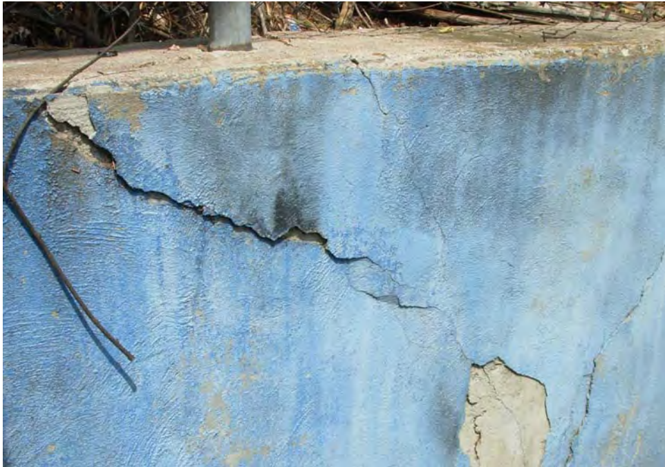
5. Spot concrete spalling of rear retaining wall
