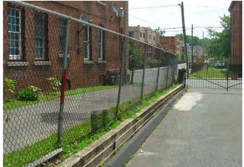
4. Wood retaining wall deterioration
