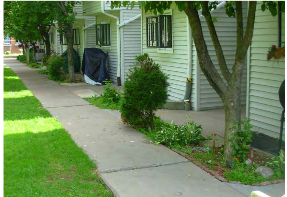
2. Concrete walkway heaving, trip hazard concerns
