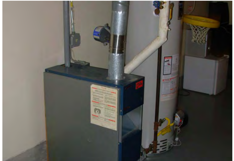
16. Typical heating boiler and DHW tank, in unit basements
