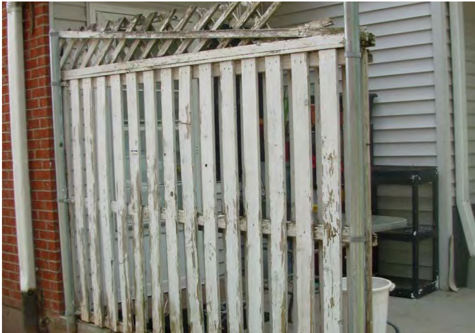
7. Wood privacy screen deterioration, to replace
