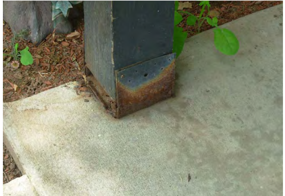
10. Entrance canopy support post deterioration observed
