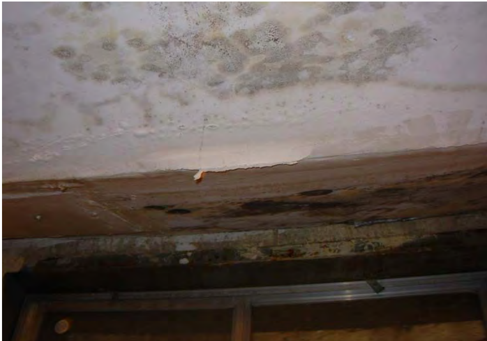
15. Leak damage from kitchen above, in basements of some units
