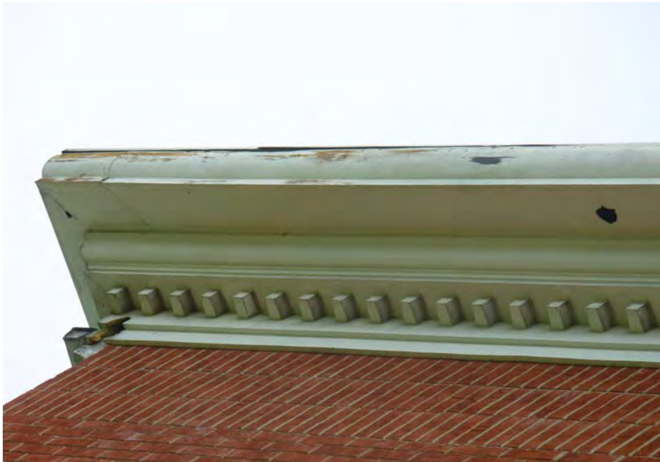
11. Soffit deterioration observed, to repair and clad with aluminum
