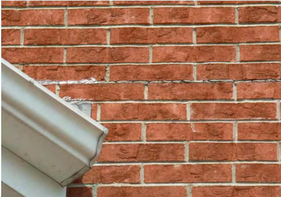
9. Brick expansion joint sealant to replace
